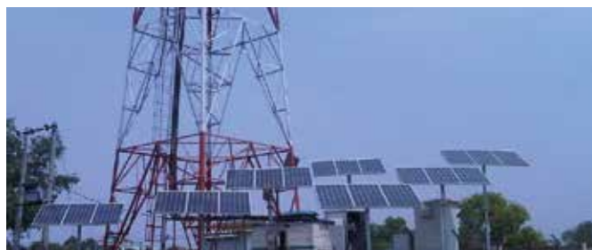
Telecom tower with AST hybrid solar solution
